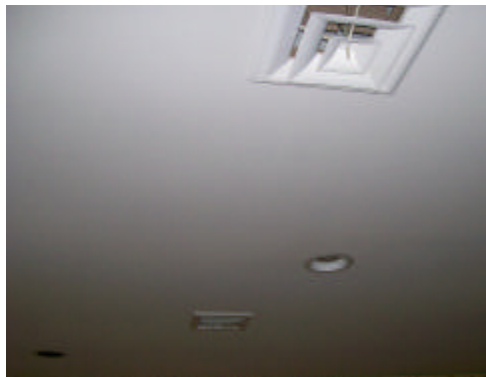
Typical “holey” ceiling
